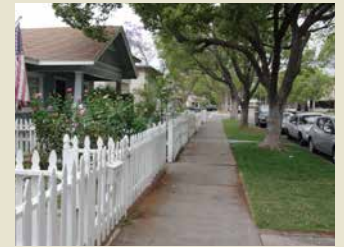
A pedestrian through zone and street furniture/buffer zone with planting, Santa Ana
