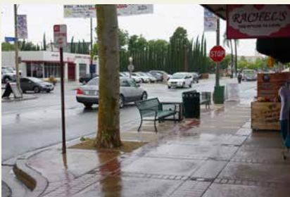
Bulb-out on the corner of North Glassell Street and Maple Avenue, Orange Plaza
