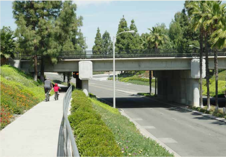
Pedestrian and bicycle underpass under railway, on Dale near Buena Park station
