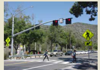
HAWK crossing installed by Caltrans outside the Laguna College of Art and Design on Laguna Canyon Road.
