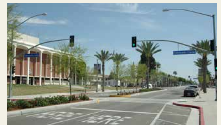
Although not raised, this mid-block crossing in Fullerton outside the City Hall features curb build-outs and different surface material
