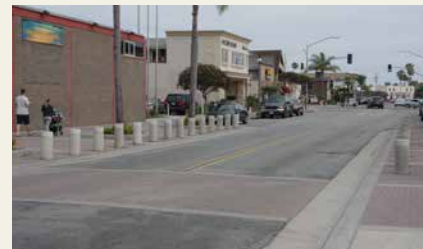
Main Street, Huntington Beach Art Center; although not a speed table, sections of raised roadway such as this can provide similar traffic calming benefits
