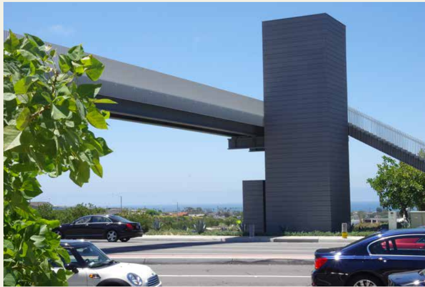
Pedestrian bridge over San Miguel Drive, Newport Beach
