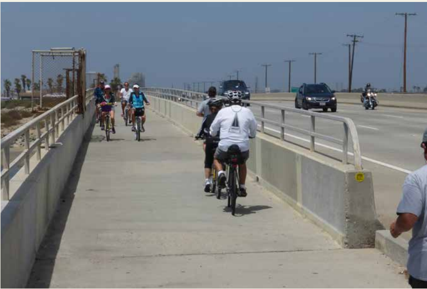
Pacific Coast Highway, Santa Ana River crossing
