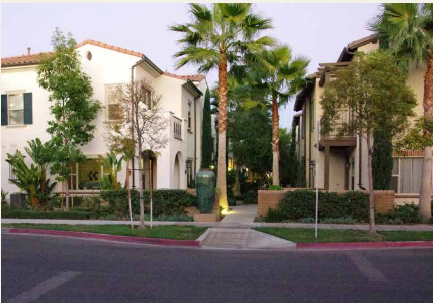
Housing in South Melrose Street, Anaheim with doors and windows addressing the street to provide natural surveillance and activity, and low walls to define public vs private areas
