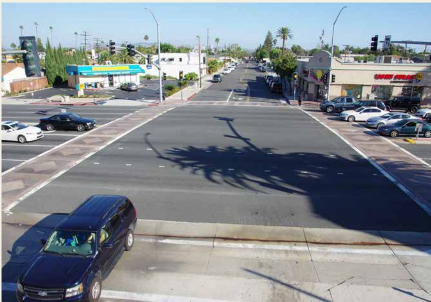
Traffic signals at the intersection of Broadway and Newport Boulevard, Costa Mesa
