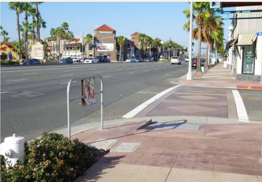
Curb ramps and detectable warning strips, Newport Boulevard, Costa Mesa
