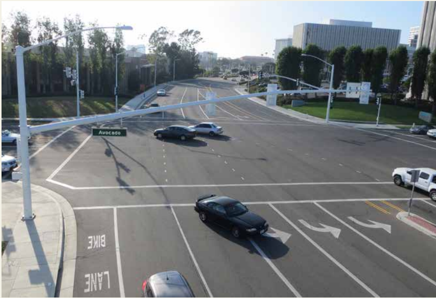
Traffic signals at the intersection of Avocado Avenue and San Miguel Drive
