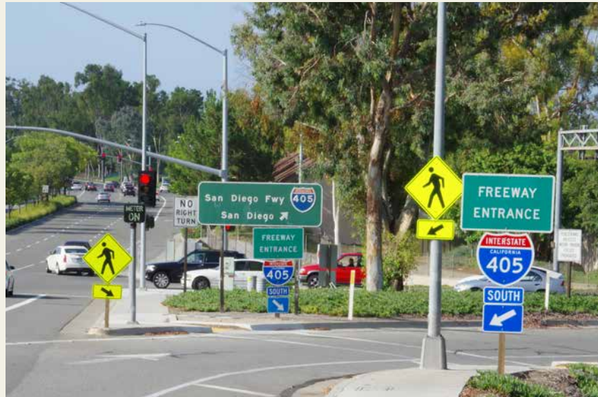
Traffic control devices, Irvine, showing how excessive signage and signage at low levels can create hinder visibility between road users
