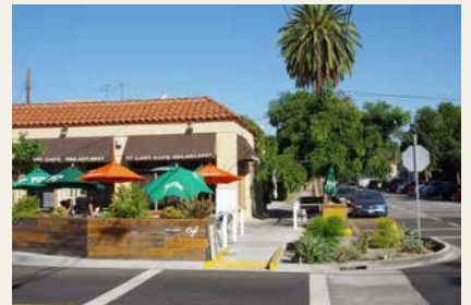
Bulb-out on the corner of Orange Avenue and 2nd Street, At Last Cafe, Long Beach
