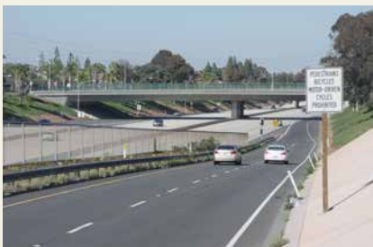
CA State Route 55, Costa Mesa, between Fairview Road and E Wilson Street
