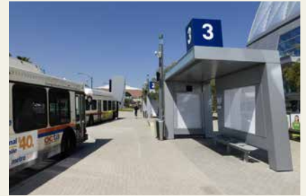
Bus shelter at ARTIC Transit Hub, Anaheim.
