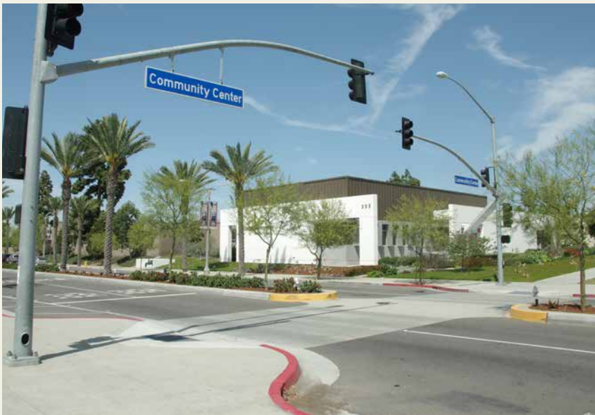
Signalized midblock crossing with bulb-outs, Fullerton
