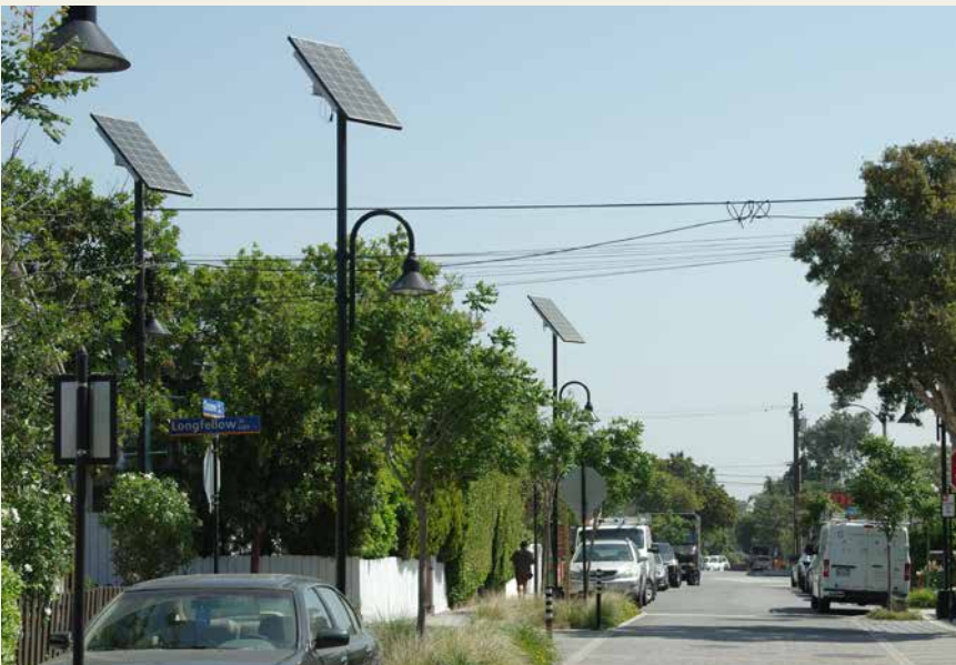
Solar powered street lights on Longfellow Street, Santa Monica
