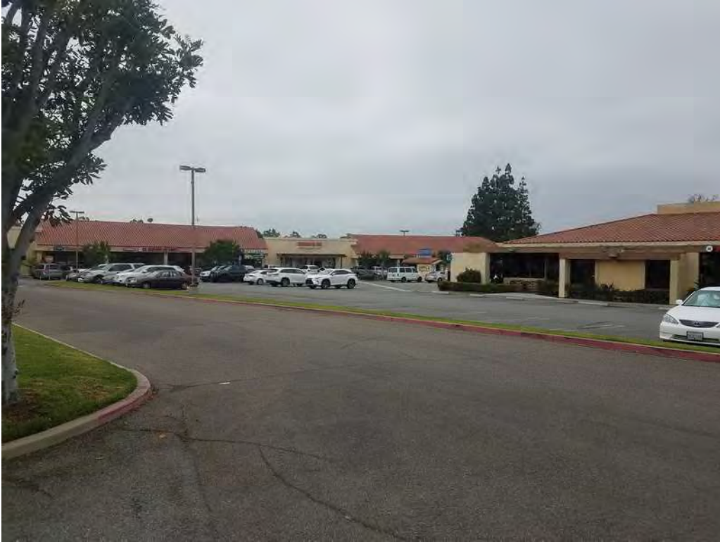
View of southeastern adjoining shopping center with open site assessment (23532 El Toro Road).
