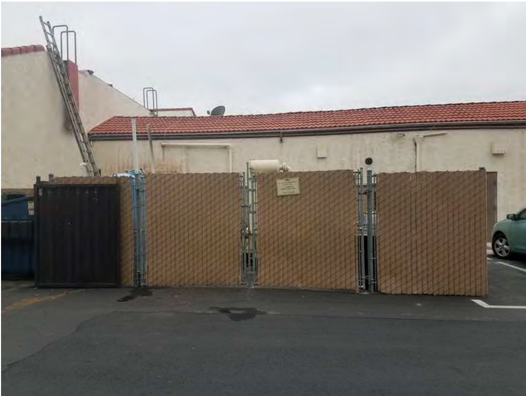
View of remediation compound at rear of former drycleaner tenant space (24601 Raymond Way).
