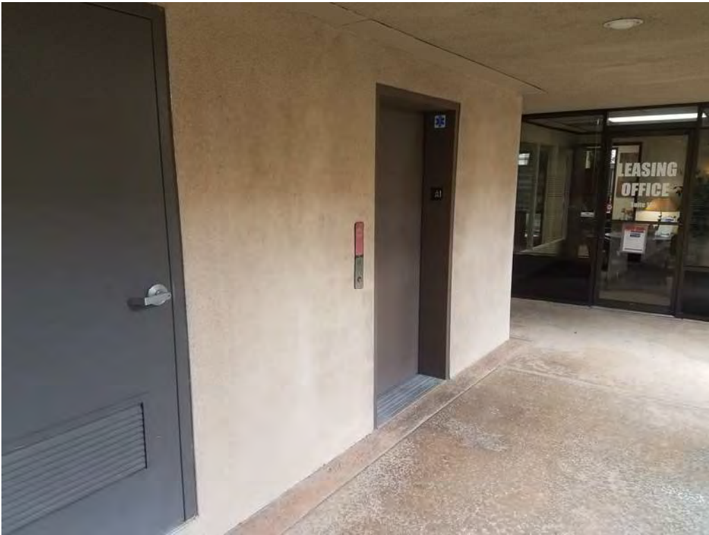
View of elevator in 23591 building.
