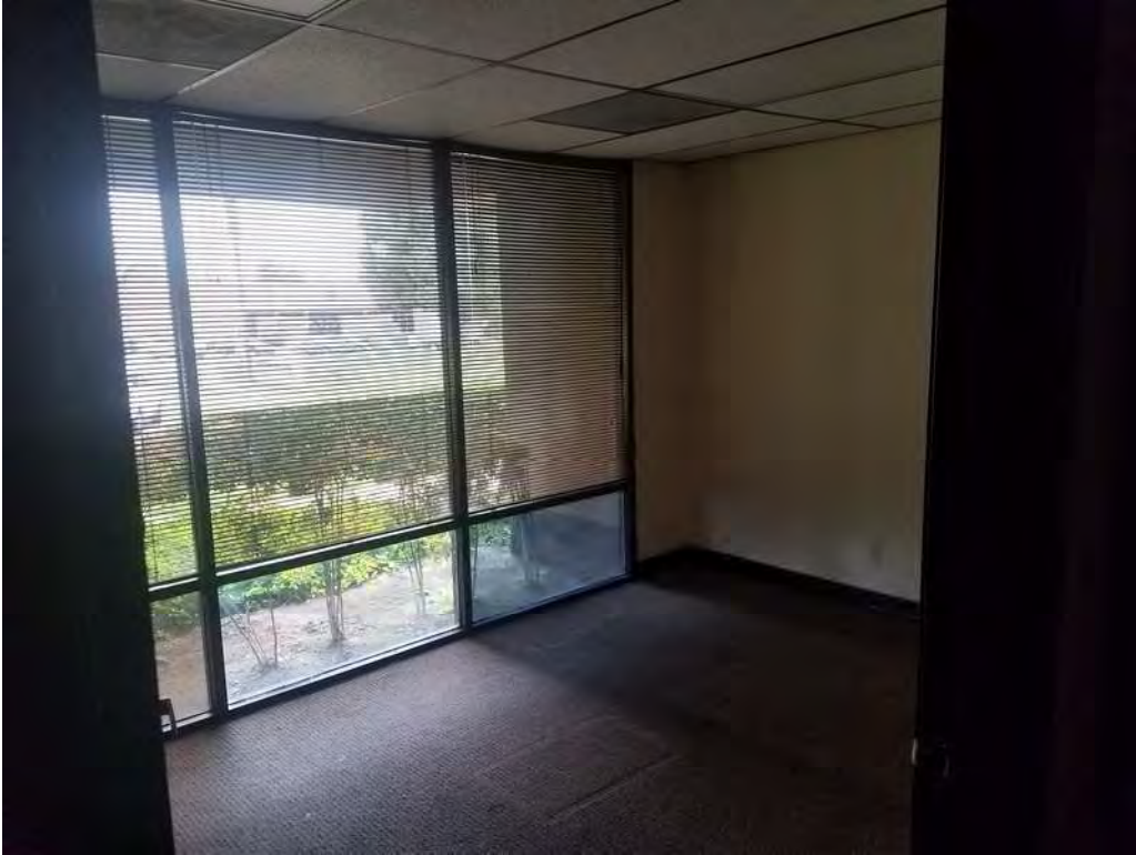
View of vacant tenant space (24551 building).
