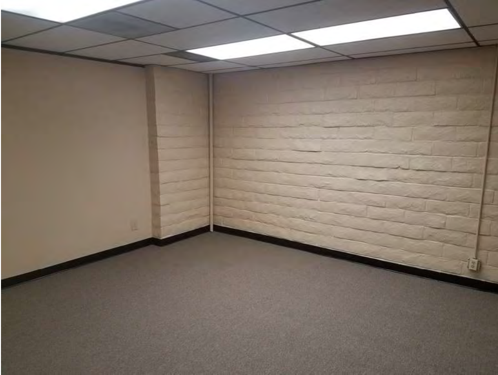
View of vacant tenant space (2451 building).
