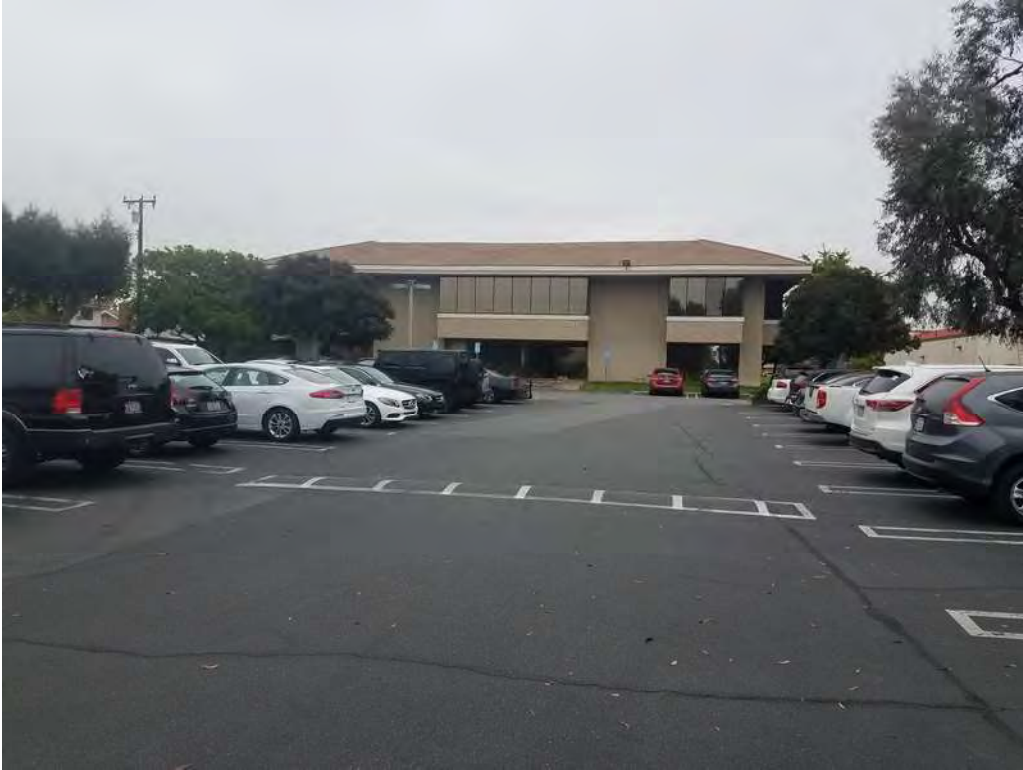
View of 23591 El Toro Road building (looking southeast).
