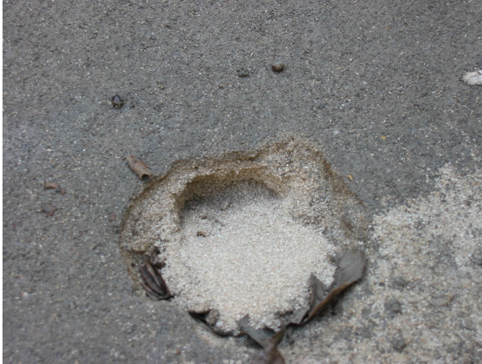
Figure 7 Formation of Clogging Crust on Filter Bed
