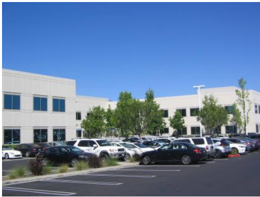
#3 EAST SIDE OF BUILDING
