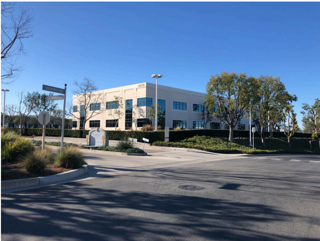
View of the southern adjoining property, facing south.
