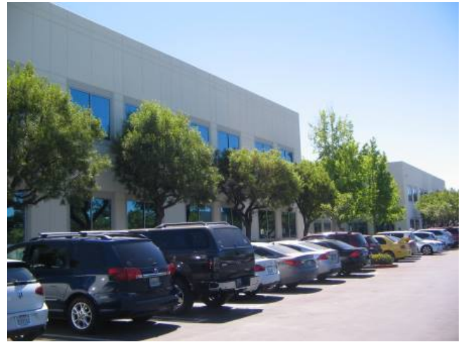
West side of building
