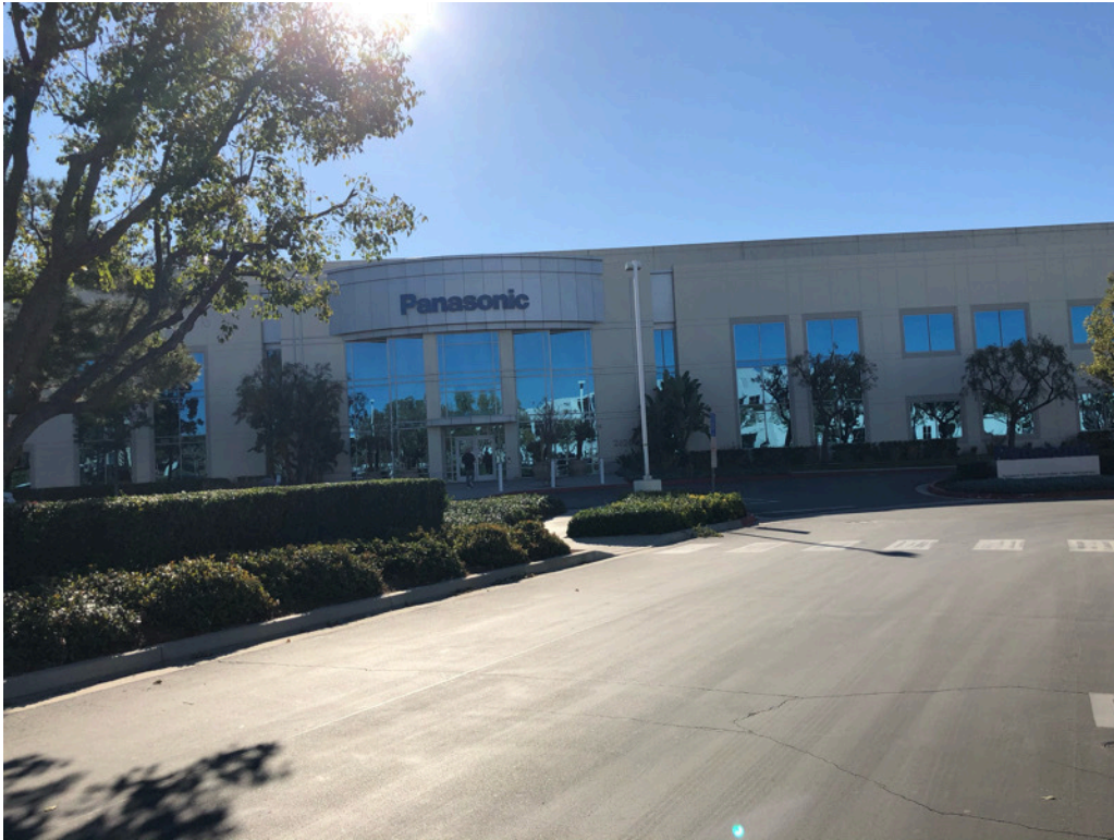
View of front main entrance to the Subject Property, facing east.
