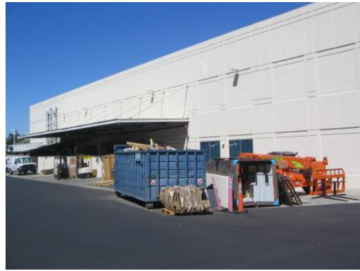
#2 SOUTH SIDE OF BUILDING
