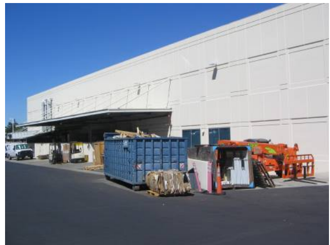
South side of building
