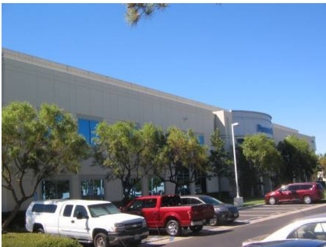
North side of building
