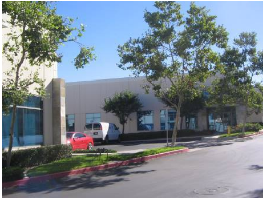
#19 ADJACENT PROPERTY TO THE SOUTH - OFFICE BUILDINGS
