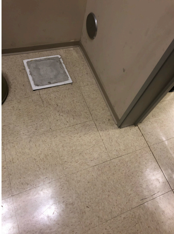
Typical floor tile in maintenance & equipment rooms.
