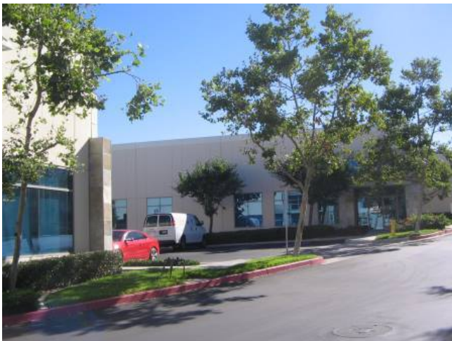
Adjacent property to the south - office buildings
