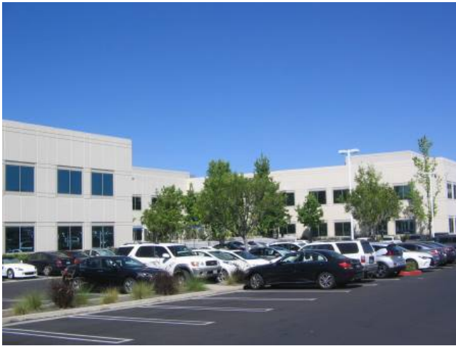
East side of building
