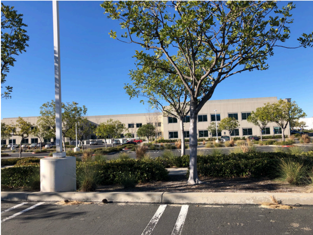
View of north side of the Subject Property, facing south.
