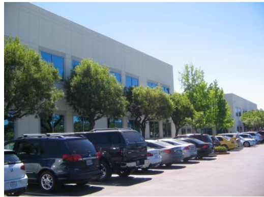
#4 WEST SIDE OF BUILDING
