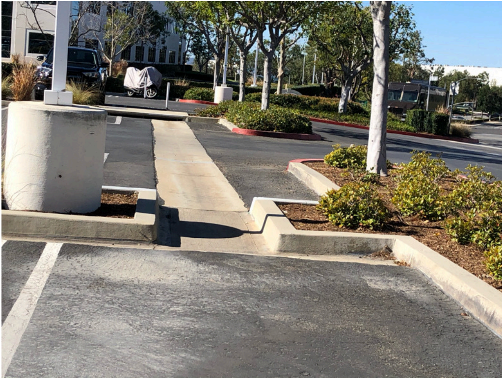
Typical drainage swale in parking lot.
