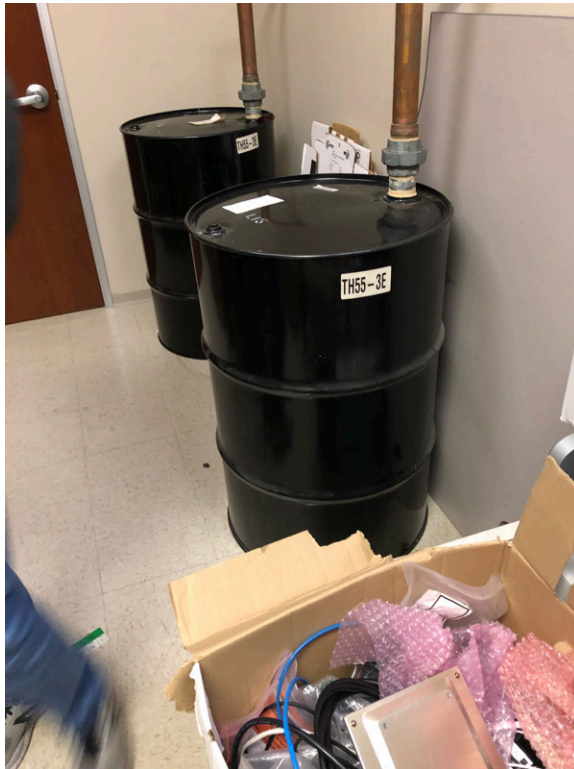
Empty and never used drums associated with the elevator equipment.
