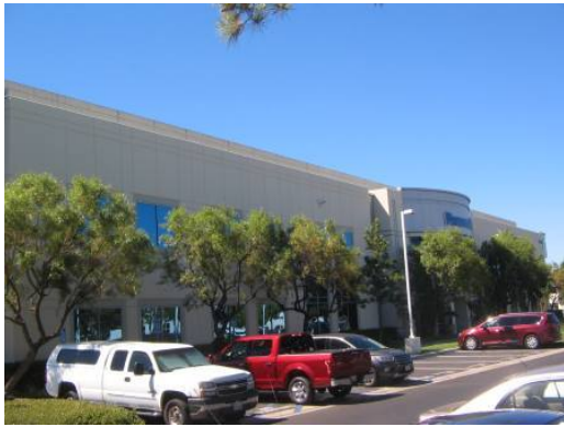
#1 NORTH SIDE OF BUILDING
