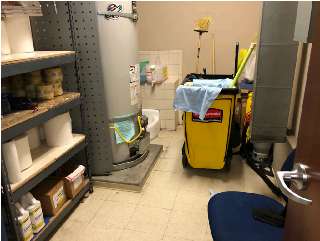
View inside janitorial closet on 2nd floor.
