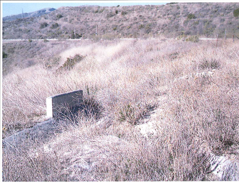
Plate 6.5-1. Overview showing the concrete drainage at Site ORA-445, facing north.
