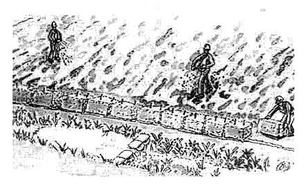
Drainage swales channel runoff around a construction site. Planting temporary vegetation on freshly graded areas, and trenching and staking straw bales and/or silt fences downslope are common techniques for preventing erosion and controlling sediment.
