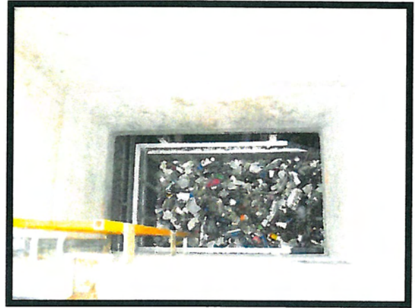
Assess Condition and Pollutant Loading Through Visual Inspection. Look at Trash & Sediment Loading.
