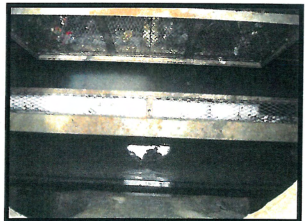
Remove Old Hydrocarbon Booms & Replace with New Ones.
