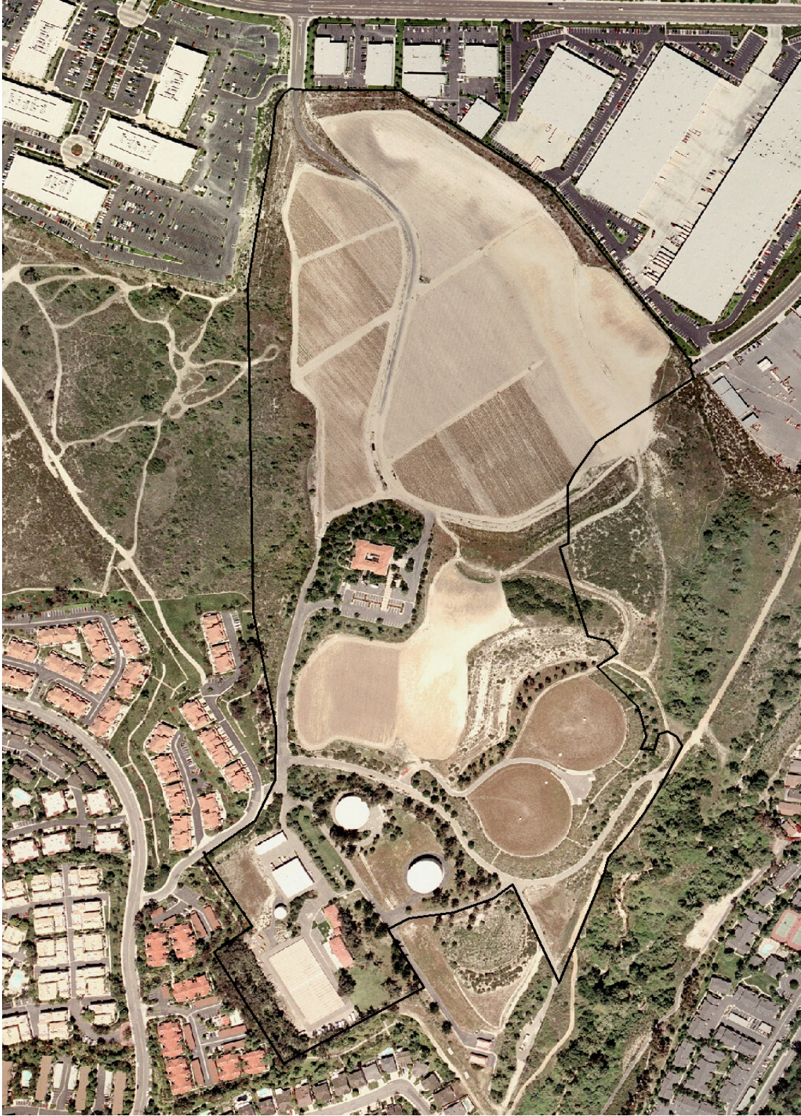
Figure 2: Lake Forest IRWD site in Orange County, southern California. Source: IRWD aerial photograph from 2005.
