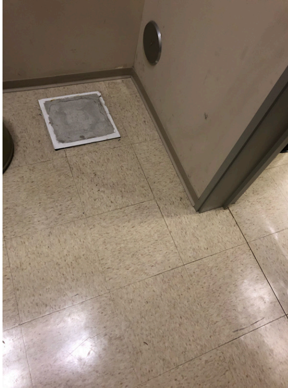
Typical floor tile in maintenance & equipment rooms.
