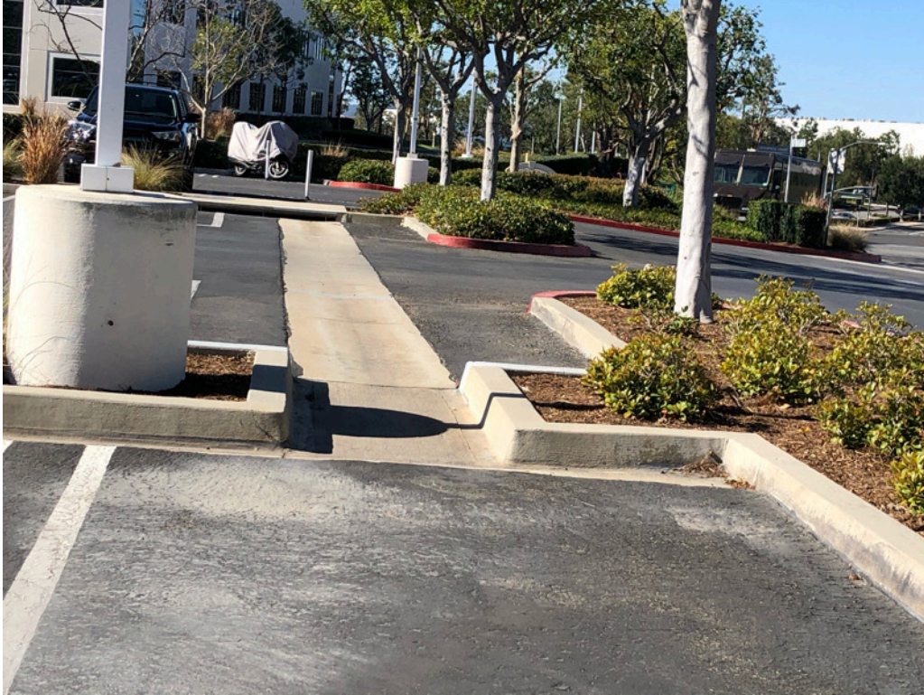
Typical drainage swale in parking lot.
