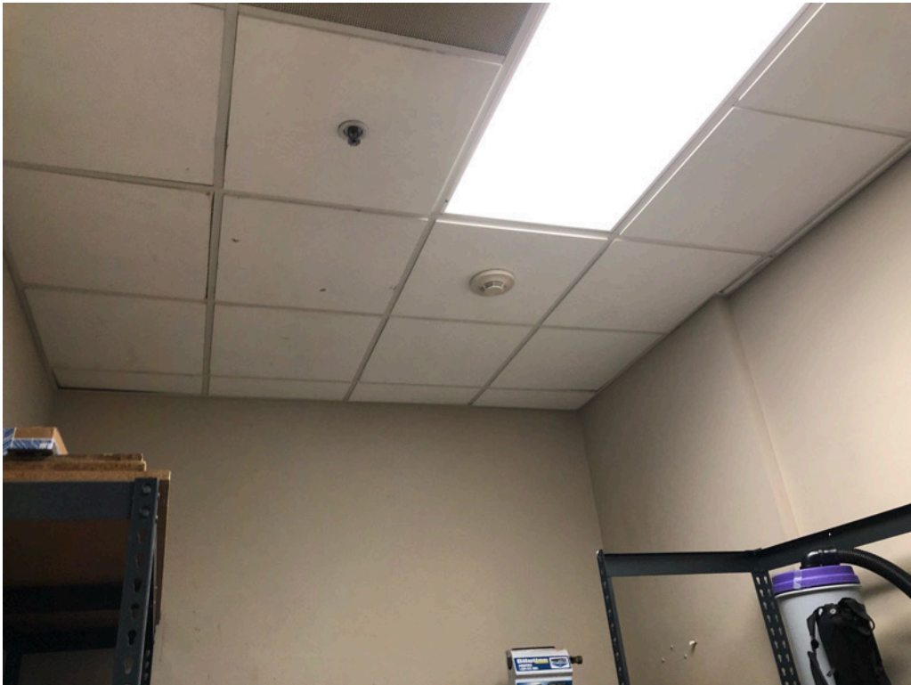
Typical acoustical ceiling panels.
