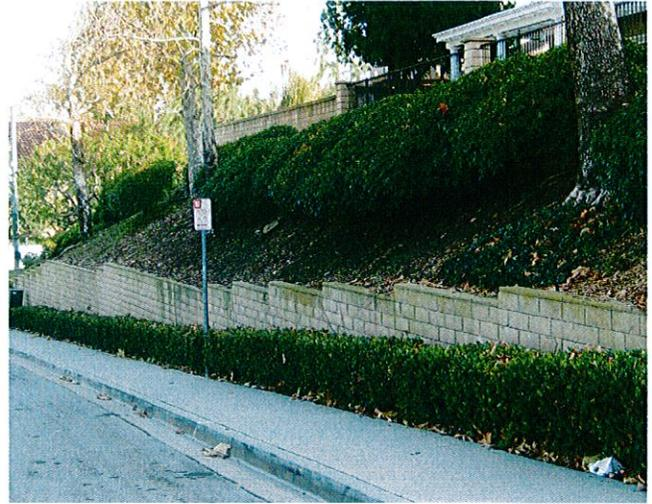
Figure 20: Retaining Wall/Slope Combination (Lake Forest)
